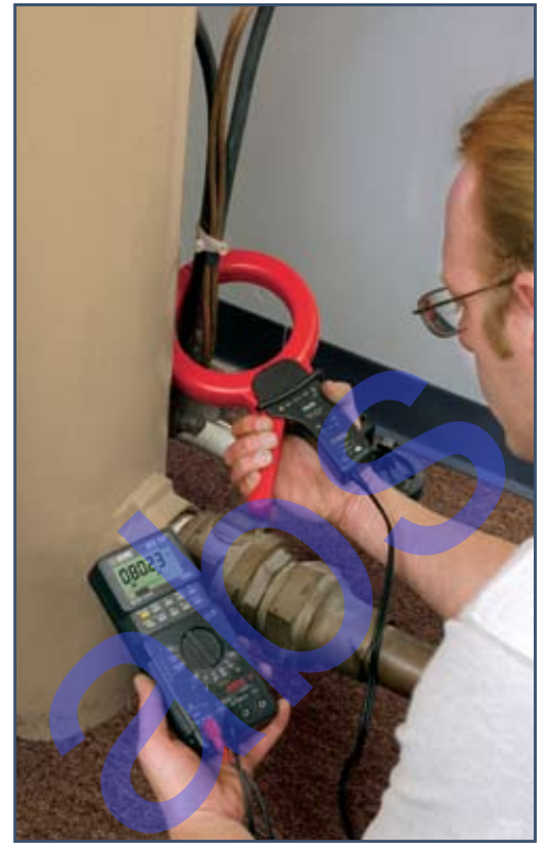
Model 2620 checking for ground fault currents
